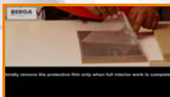
Step 15 : Kindly remove the protective film only when full interior work is completed.
