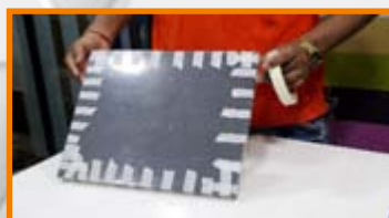
Step 13 : Time taken for the setting of the glue is 10 to 15 hrs
